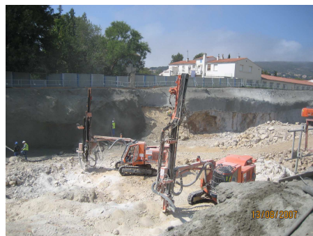
Parking VINCI La Ciotat, 2 foreuses hydraulique assurant 400 m 3 /j.
